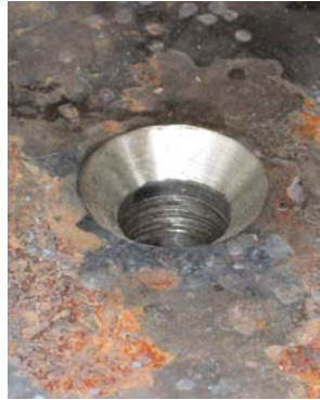
#2 Hook plate holes are countersunk.
