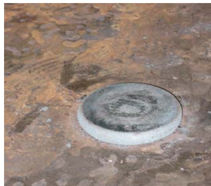
#7 Properly punched rivet
