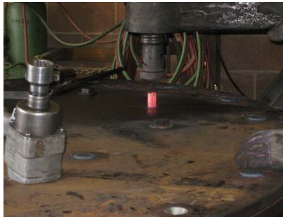
#5 Hot rivet is inserted from bottom side.
