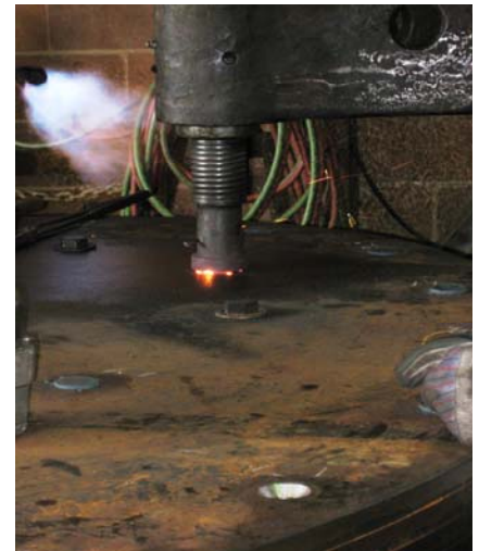
#6 Rivet is punched using the riveting machine.
